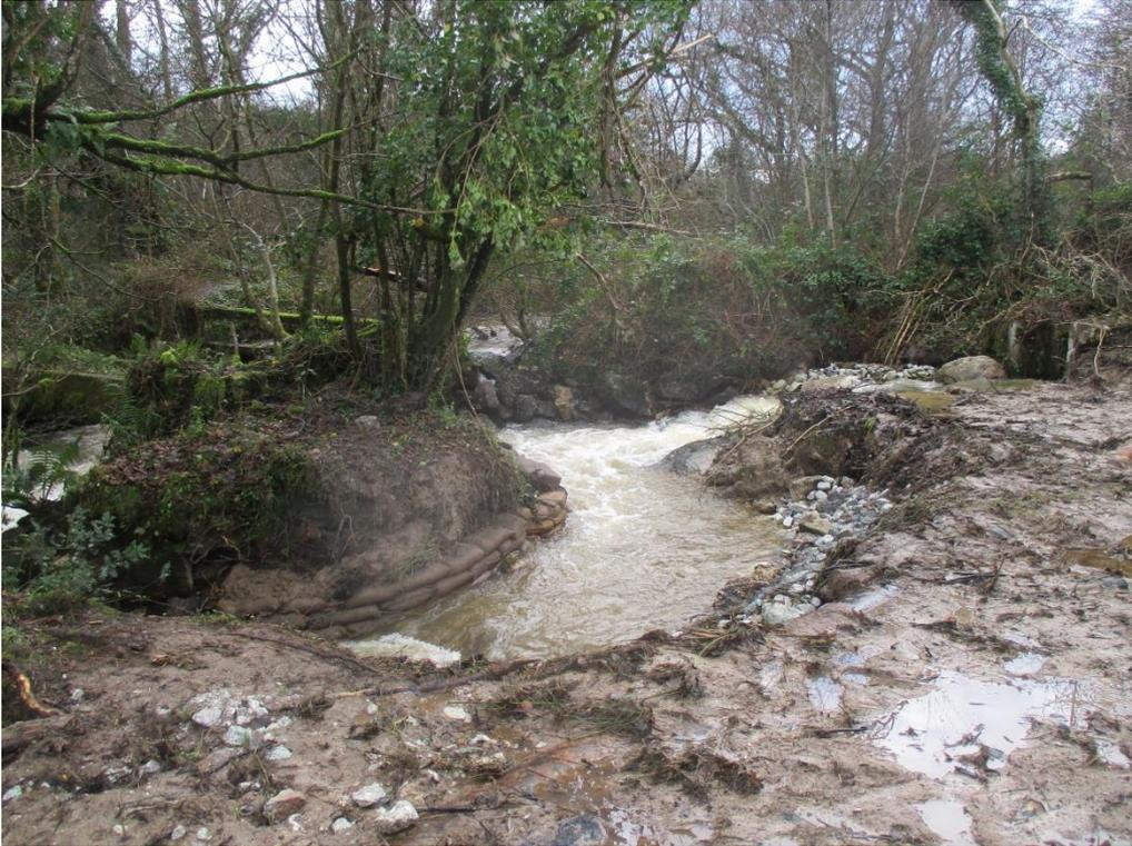
Recently works have been carried out near Cam Bridges weir. It is hoped that the channel to the right will serve as a fish-pass.
